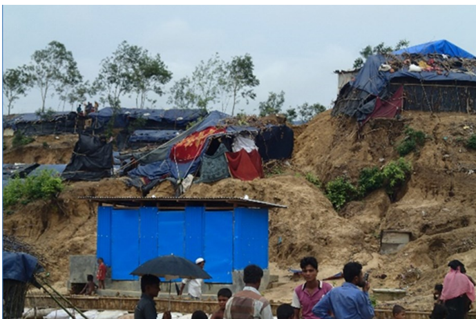
Damage caused by Cyclone Mora at Balukhali Makeshift Settlement. ©IOM 2017
